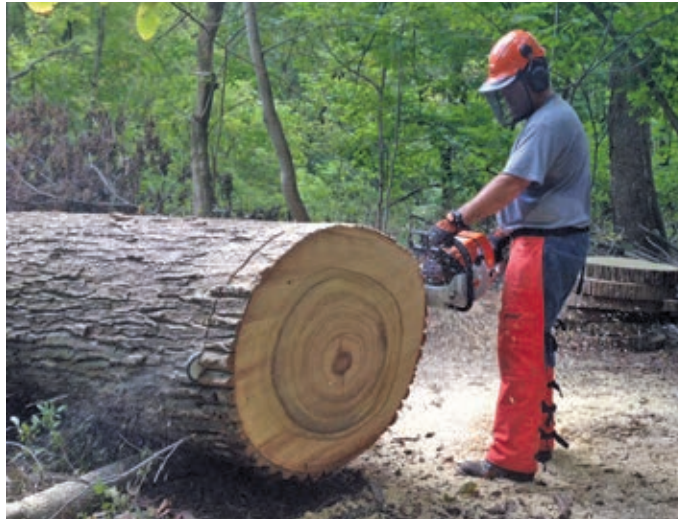
A Habitat and Trails volunteer cuts 'cookies' from 108" diameter poplar tree on the L'Hirondelle Trail that can be placed on muddy portions of a hiking trail. Photo: Jeffrey Budnitz
